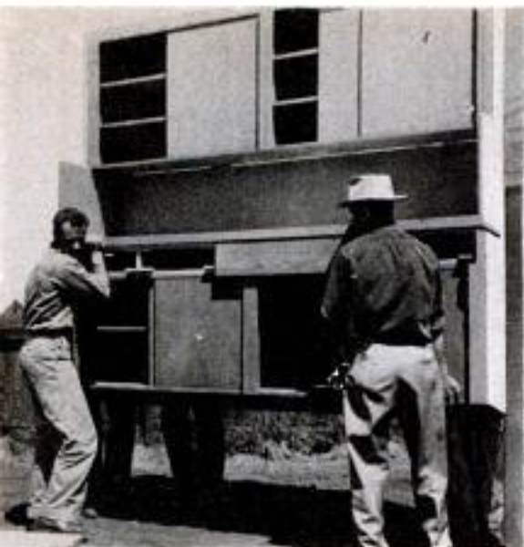
Prebuilt kitchen cabinet wall made of hardwoods is moved into a new May home
